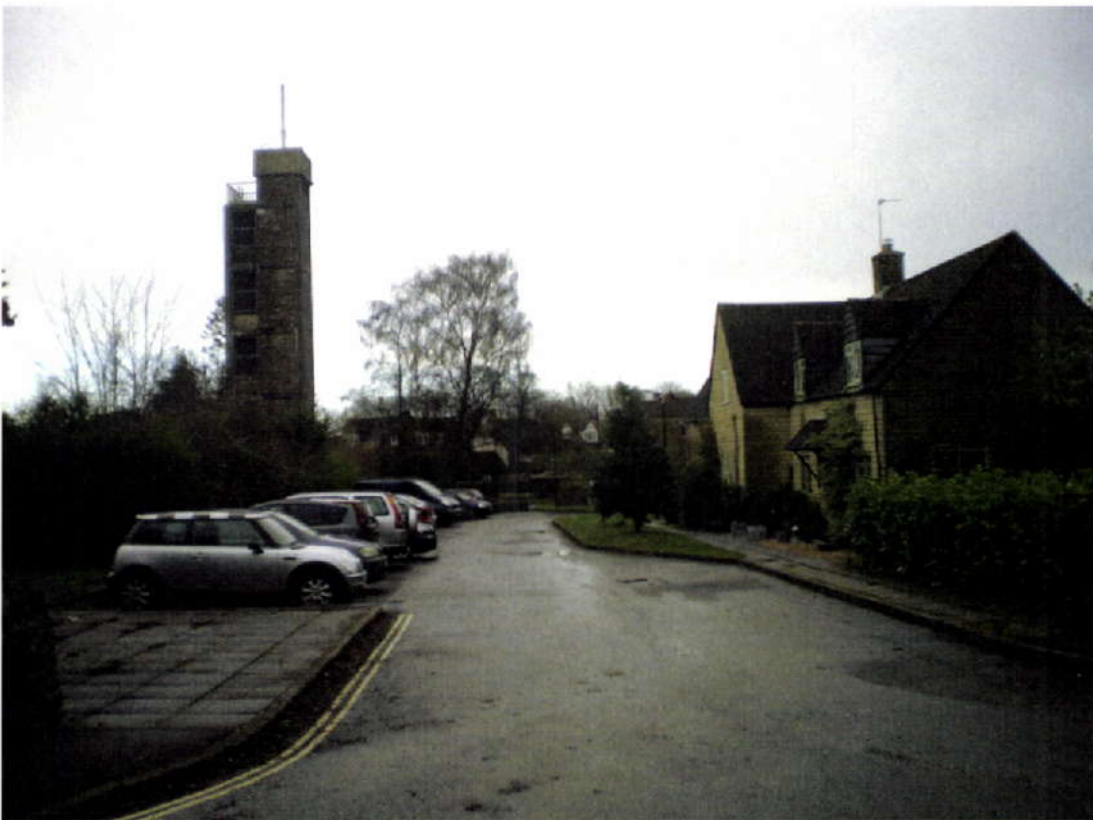
Below: Site Entrance
